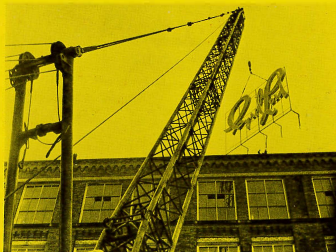
Raising a 30 foot sign 100 feet high, on the Cyril Lord Textile Factory near Oldham presented some interesting problems to Astley installation engineers. Our front page shows this sign in action at night.
